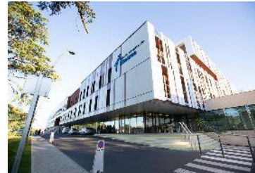
Centre Hospitalier de Libourne, France
